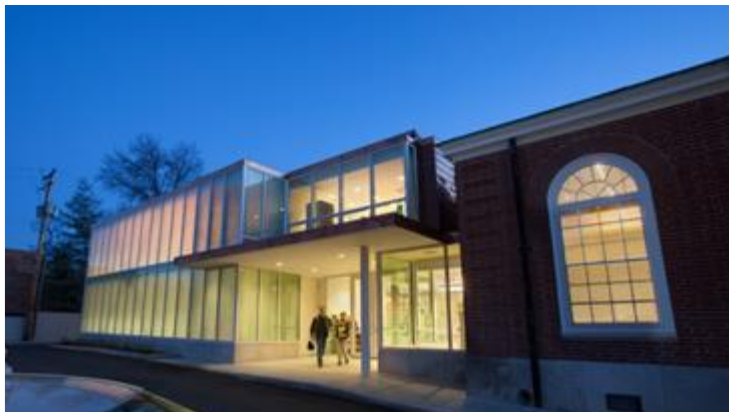
The completed addition
